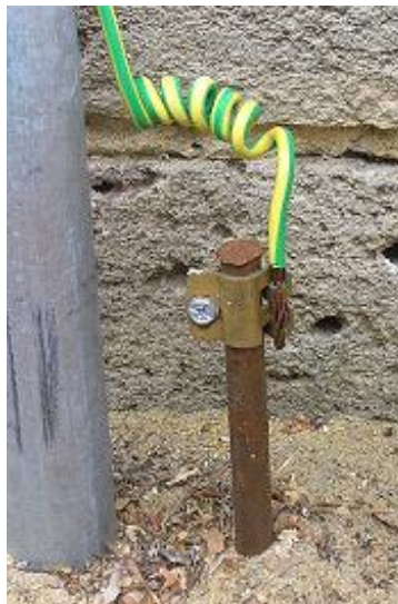
Figure 5.32 Earth ground implementation
